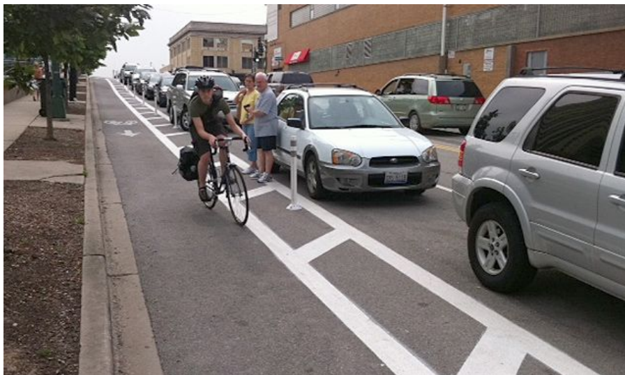
Figure 14. A car protected bike lane with additional protection from bollards. Source:
