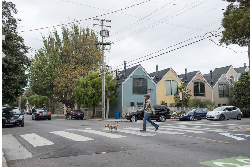
Figure 16. A raised crosswalk. Source:
