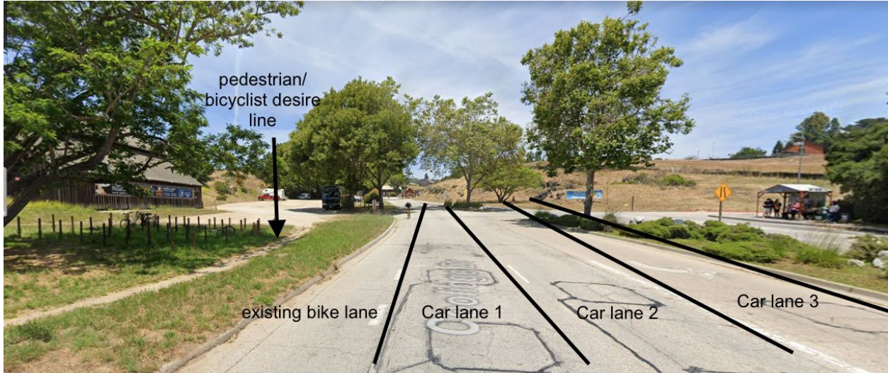
Figure 5.1.5: The “before”: current situation of Coolidge Dr with 3 car lanes and desire line for nonexistent pedestrian walkway & northbound bicyclists
