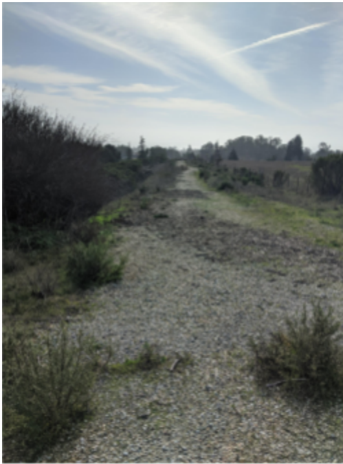
Figure 3.2.1: Existing Utility Corridor conditions
