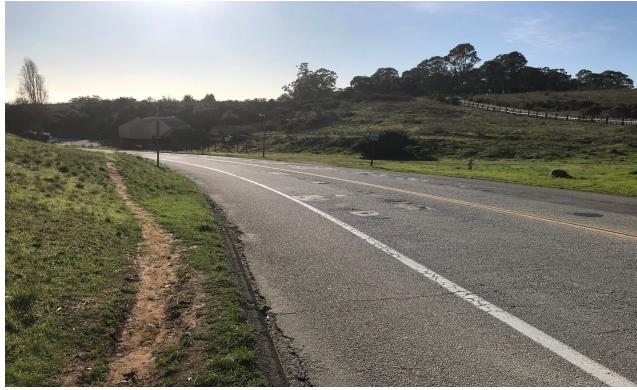
Figure 3.2.3: Desire lines created by pedestrians on Coolidge Dr. due to the lack of sidewalk and pedestrian infrastructure.
