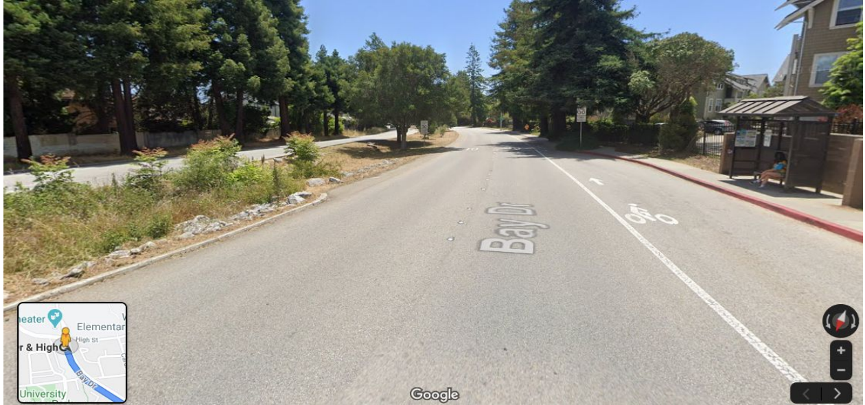
Figure 16 Looking Southbound, two car lanes, bus loading zone placed inside of unprotected bike lane
