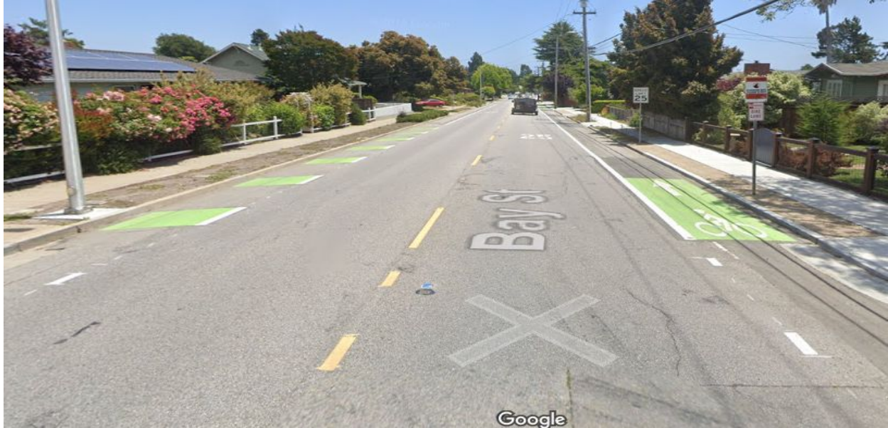
Figure 24 Looking Southbound, one car lane in each direction, painted bike lanes without protections for turns (conflict zones)
