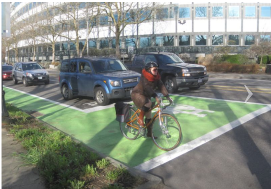
Fig 12. A cyclist waits at an intersection in a green bike box Source (NACTO, 2014)
