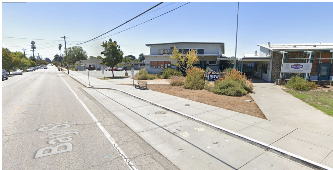
Figure 32 Unprotected bike lane that is also within a bus loading zone in front of Bay View Elementary
