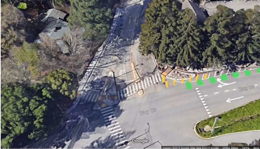
An aerial view of the corner of Bay Dr & Meder St with flexible bollards.
