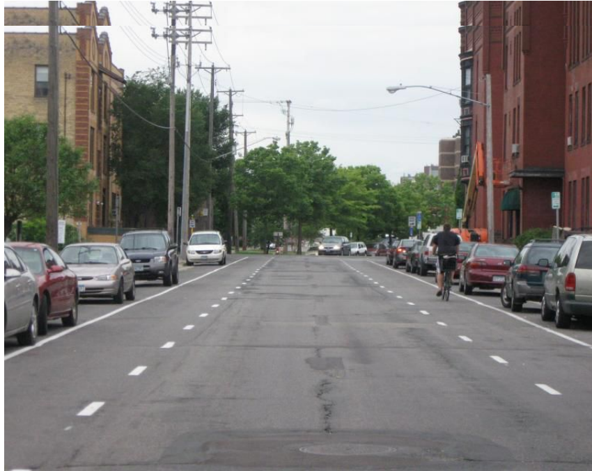
An advisory bike lane in Minneapolis' Elliot Park. This design need not remove parking.
