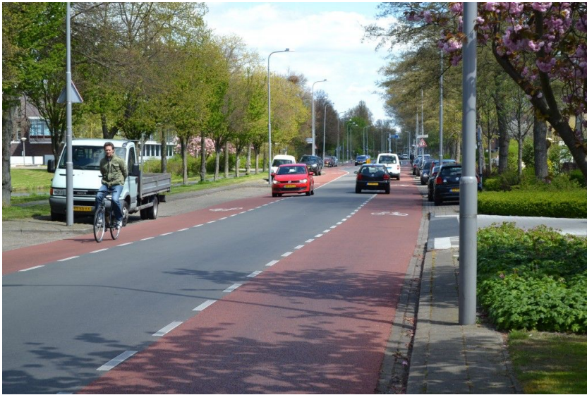
Advisory bike lane in the Netherlands (Greater Auckland). Paint can be used to enhance visibility for cyclists and to keep cars alert.
