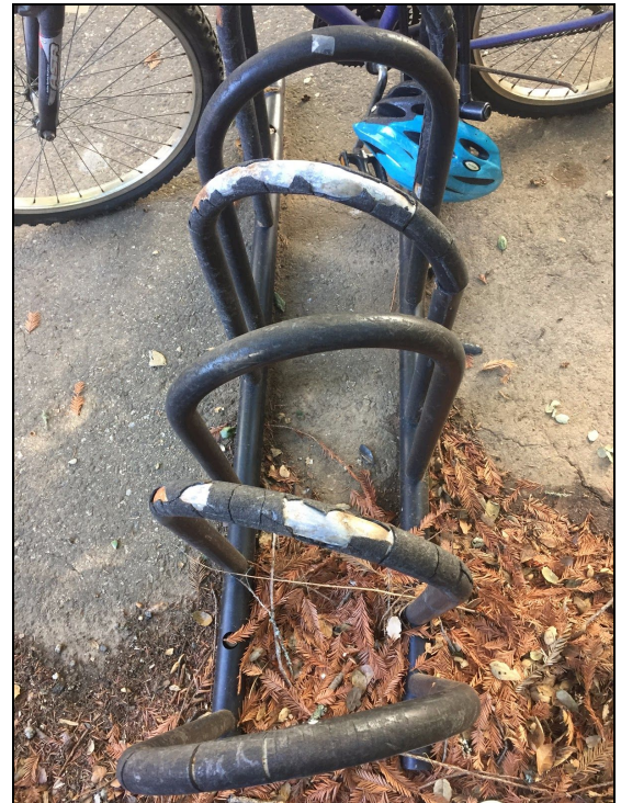
Figure 12: Example of a Cracked Rack
